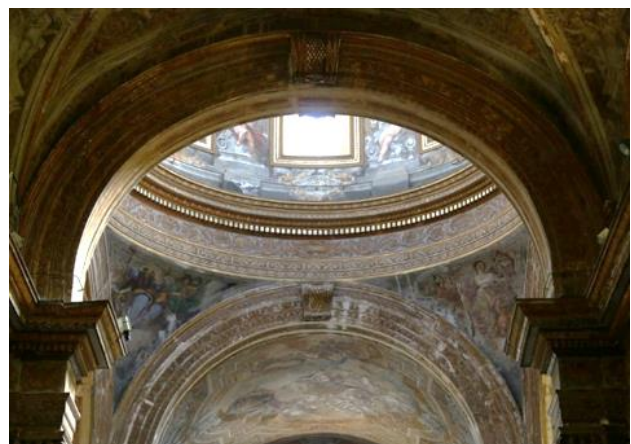
Figures 6 and 7. Naples, Santa Caterina a Formiello Church. The right side of the transept, the bell tower and the massive dome. Below, an internal detail of the crossing.
