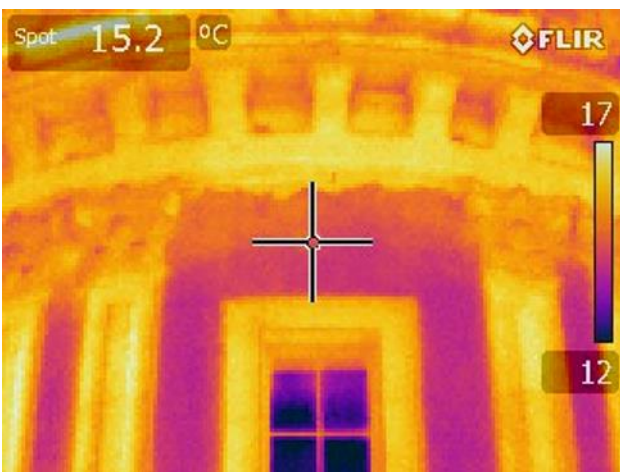
Figure 13. Santa Caterina a Formiello Church. Thermal photography of a span of the drum (R. Amore and M. Facchini, DiARC MLab, 2019).
