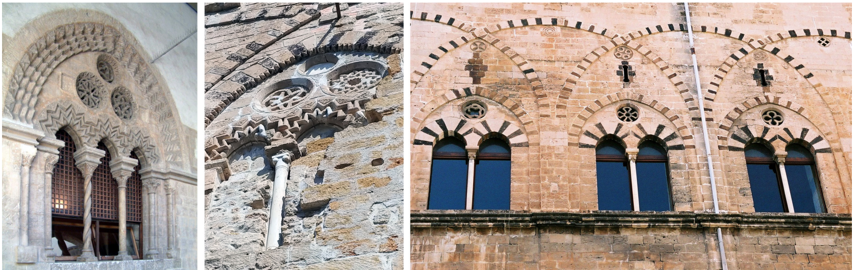
Fig. 9-11: Comparison between the windows of some 14th century palaces in Palermo. Chiaramonte palace on the left, Cefalà palace at the centre and the series of windows at the main floor of palazzo Sclafani on the right (photos by the autor).
