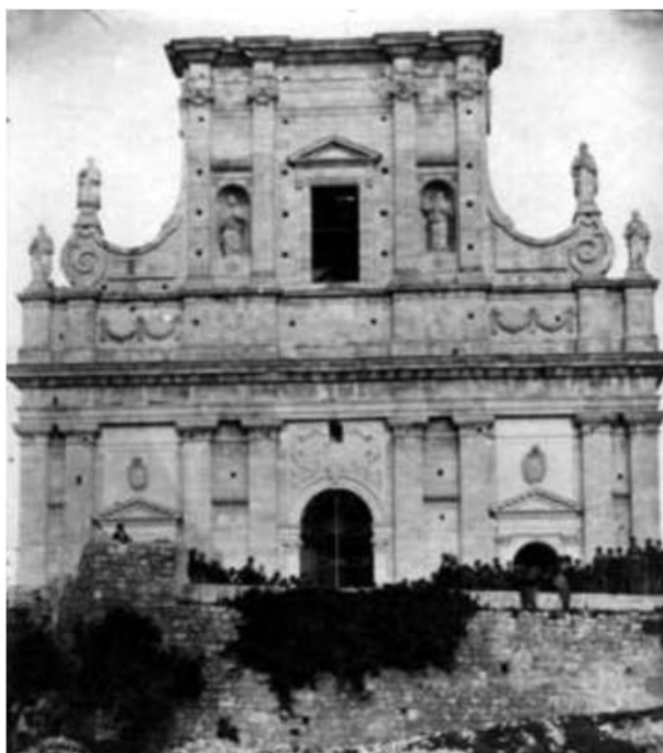
Fig. 5: Santa Maria delle Stelle church with its façade raised up to the level of the second order; the construction site has been interrupted since 1884, Diocesi di Ragusa, Archivio Parrocchiale della chiesa di Santa Maria delle Stelle, f. Globo II.
